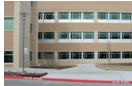
Chemistry Building - ribbon windows
