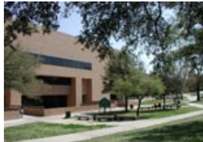
General Academic Building - west facade
