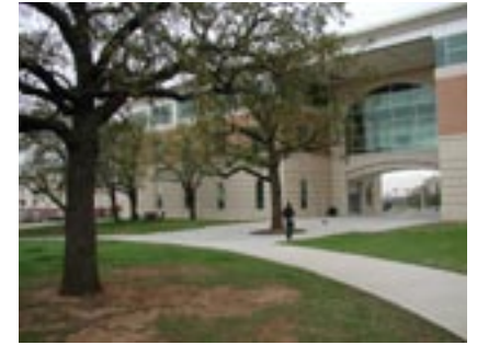
Gateway Center - east facade
