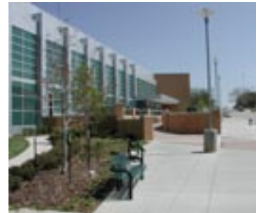
Student Recreation - south facing curtain wall and metal panels.
