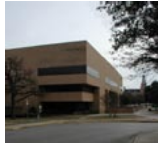
General Academic Building - west facade
