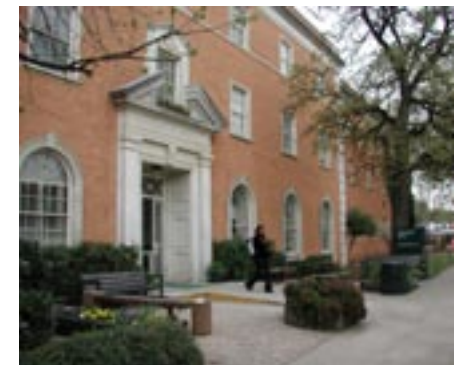
Windows in the base or ground floor are often differentiated by arches, ornament or other design features.
