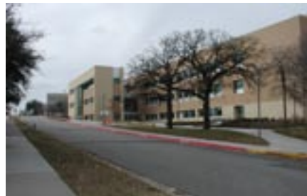
Chemistry Building - street edge condition
