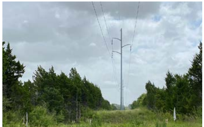
▲ Overhead electrical powerlines along on the campus perimeter. (Source: Page)
